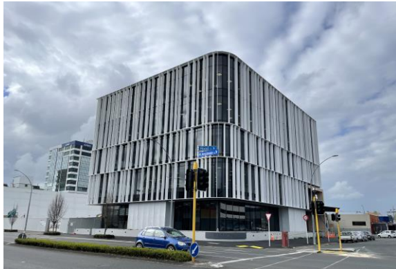
Progress of the first building at Union Square, Angelsea and Hood Streets.
